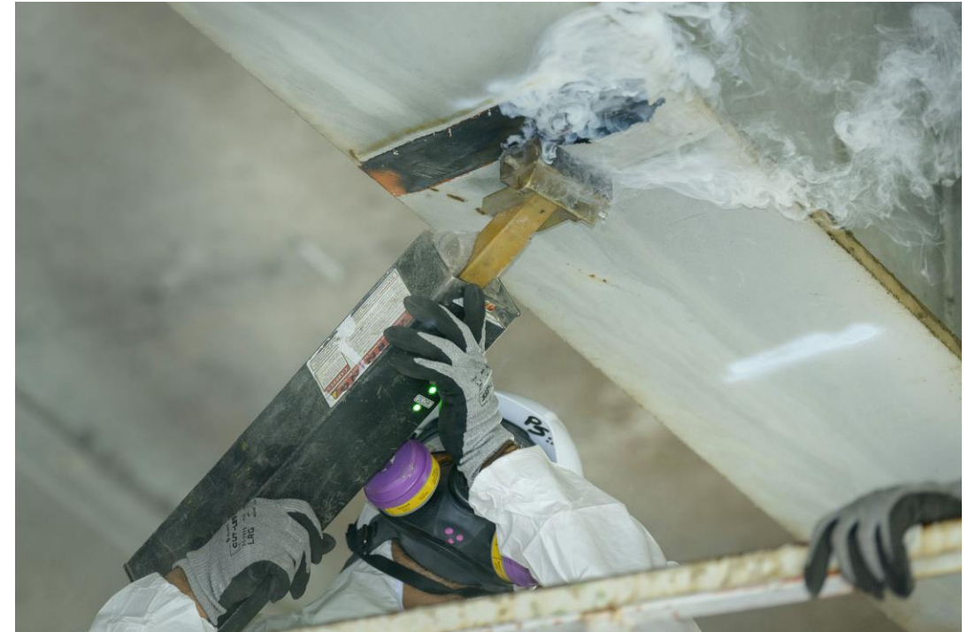
Crews remove lead paint from I-5 bridge supporting structures
