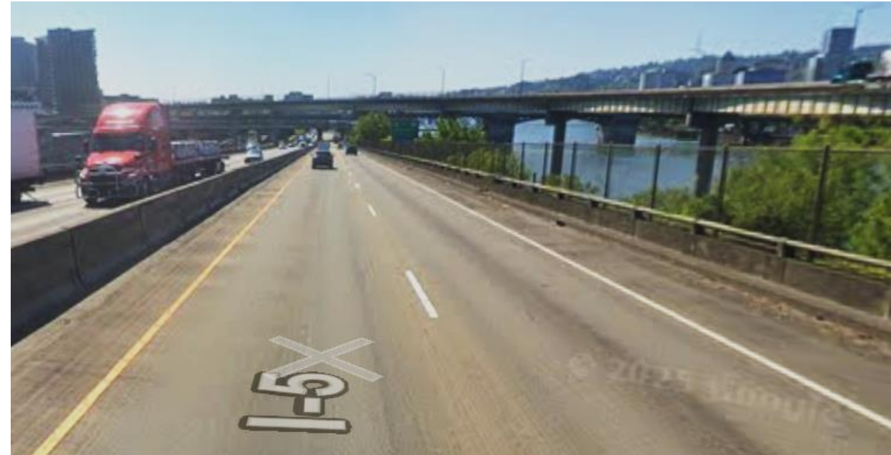
Google Street View: Driver's perspective travelling on I-5 SB through planned work area
